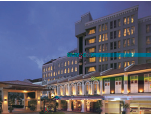
Existing Village Hotel Albert Court
